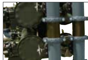
Optional condenser set up with victaulic coupling
